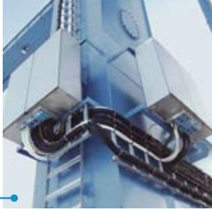
A Roxtec CF 32 transit has two openings and can accommodate several cables in a small space. Here, installed in the side of a power supply cabinet.
